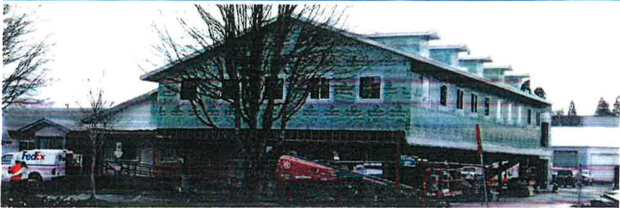
Barton County Avery Complex, Second Floor Addition, Construction progress
